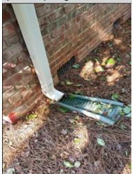
The gutter extension on the right side of the house was not sloped to drain away from the foundation. Direct drainage to the foundation and cladding from the gutter system can result in water penetration into the foundation area and foundation deterioration. A licensed general contractor should be consulted for a complete evaluation of the gutter system to reduce overflow and to make necessary repairs.
