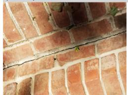
The masonry steps are in need of repair. The steps have rotated or moved away from the foundation. The crack should be caulked to prevent water penetration and further movement. A licensed general contractor should be consulted if the crack size increases.
