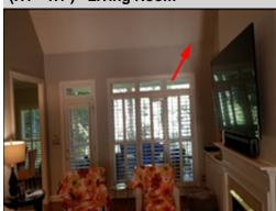
Stains on the ceilings indicate a history of a leak. At the time of the inspection it was not possible to determine if the condition was due to an active or past occurrence. Further investigation by a repair specialist and owner disclosure is recommended. Refer to the XXX section of the report.
