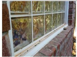
The sill on the glass block window is sloping towards the house and will pool water. It should slope away from the house to shed water. Pooling of water can cause wood rot and deterioration. A licensed general contractor should be contacted to review and repair.
